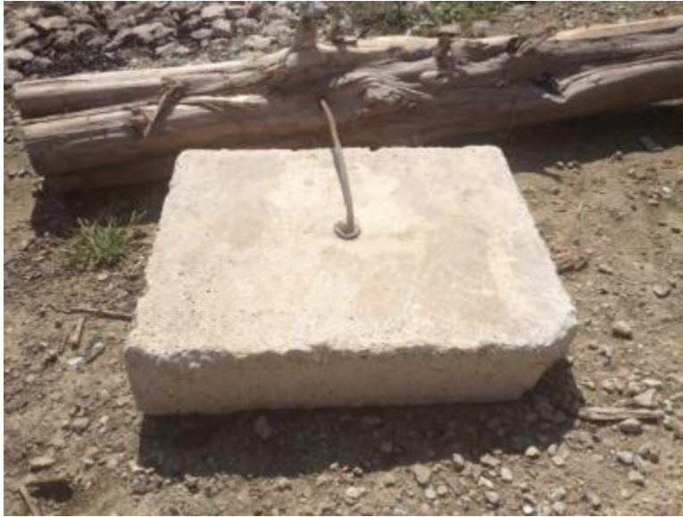
Figure 1.7: Larger concrete anchor made by contractors.
