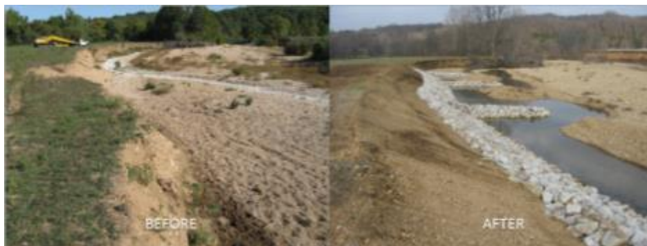
Figure 2.10: Pictures of streambank before and after completion of stabilization project 42-54-10.
