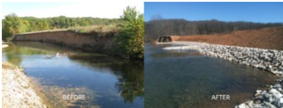
Figure 2.9: Pictures of streambank before and after completion of stabilization project 42-54-09.
