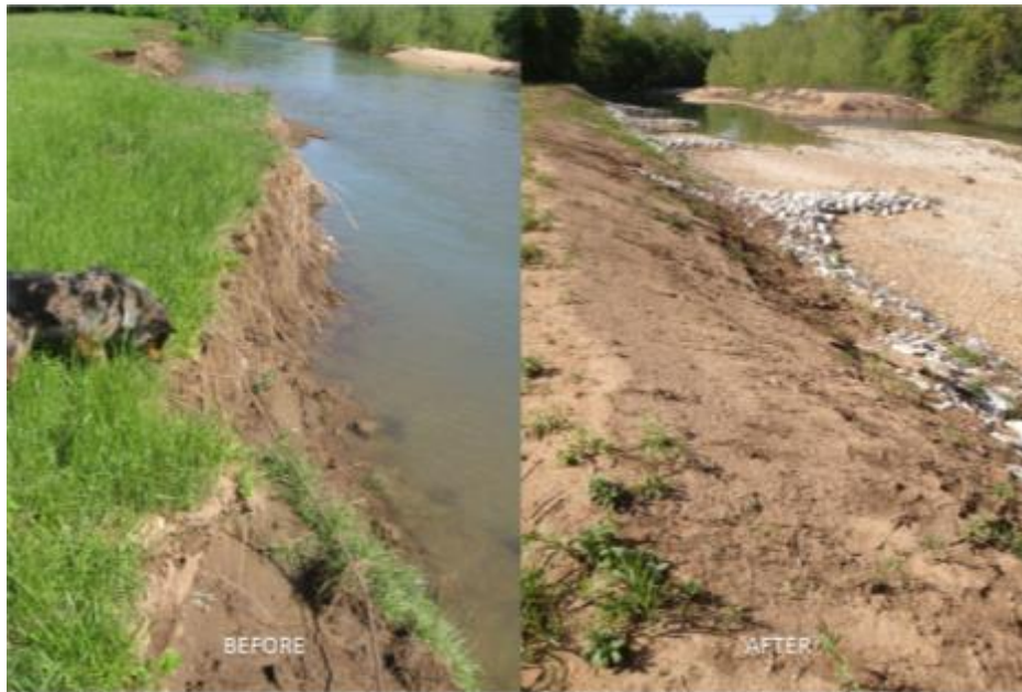
Figure 2.6: Pictures of streambank before and after completion of stabilization of project 42-54-02.
