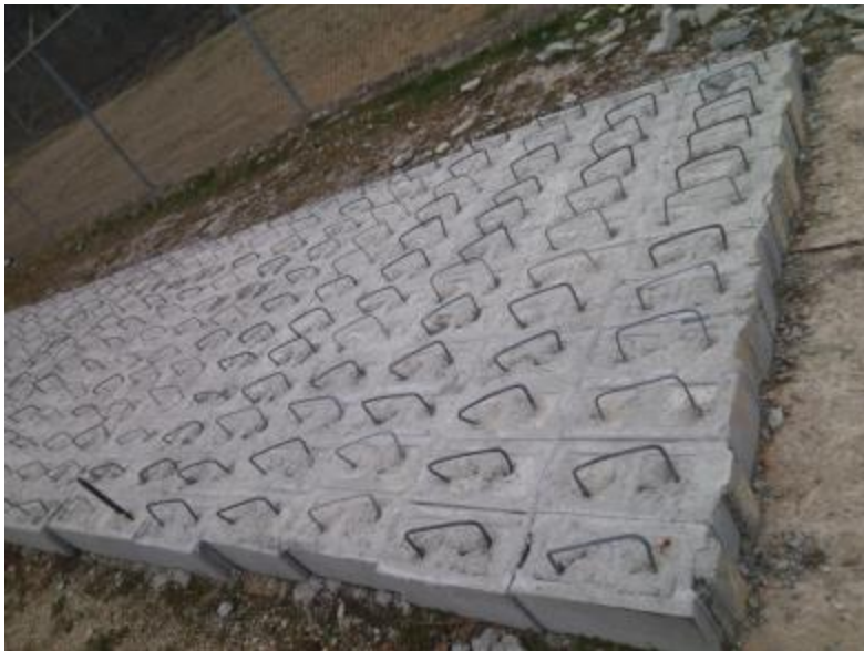
Figure 1.5: Field of finished anchors.
