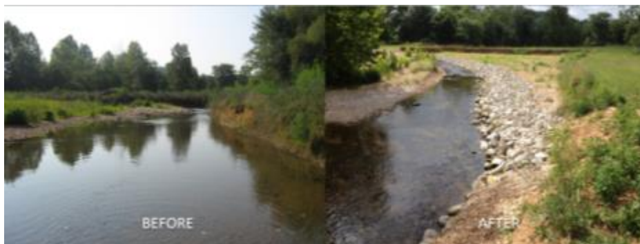
Figure 2.11: Pictures of streambank before and after completion of stabilization project 42-54-11.
