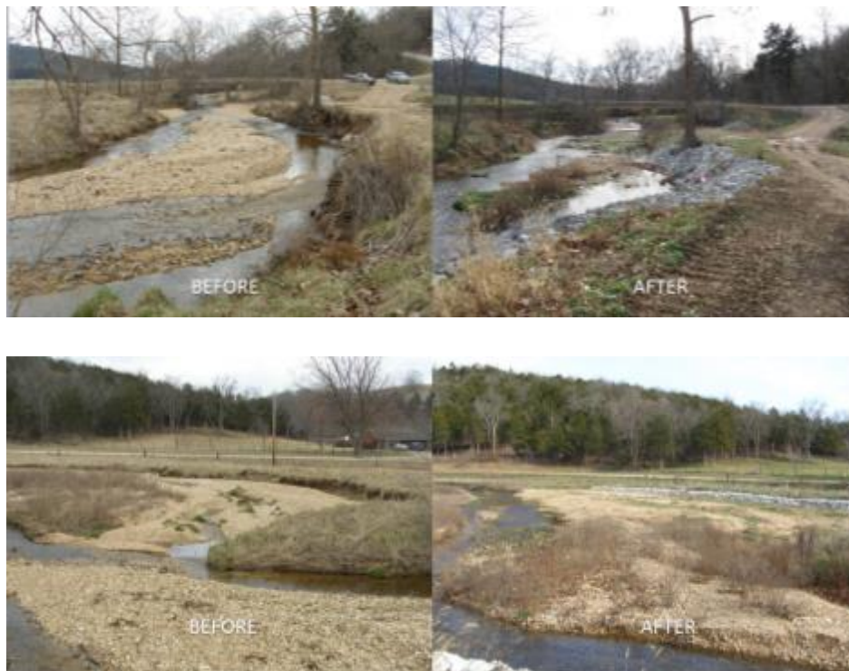
Figure 2.8: Pictures of streambank before and after completion of stabilization project 42-54-04.
