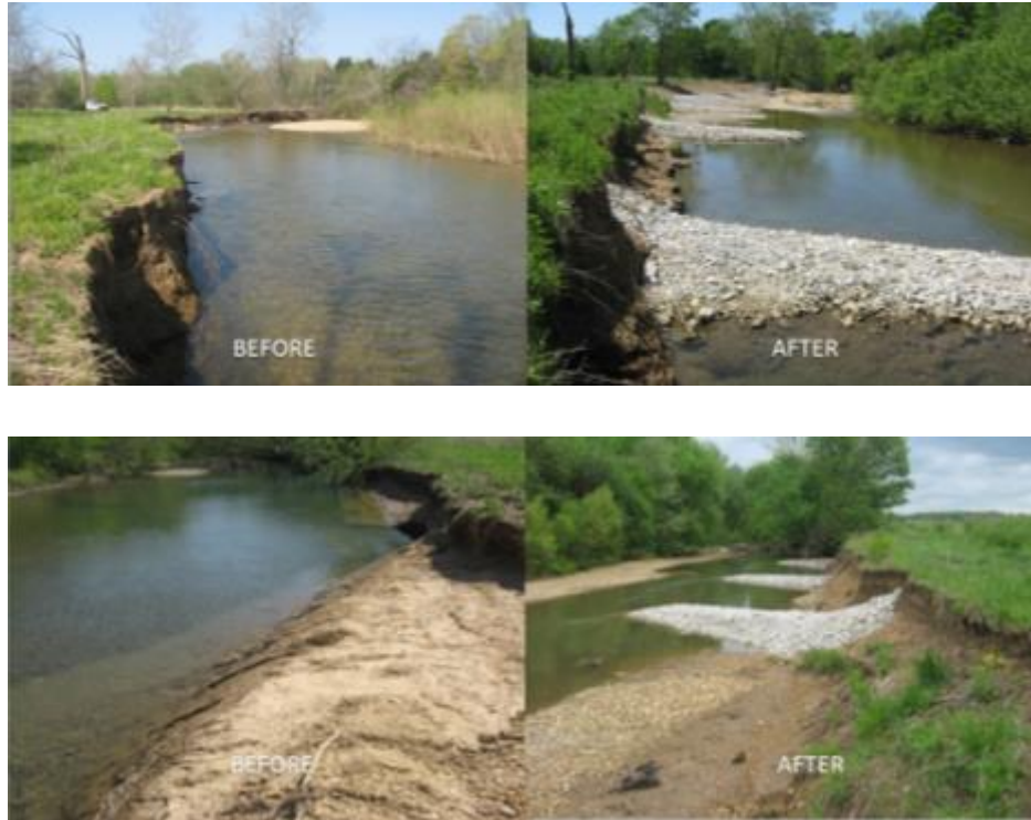
Figure 2.7: Pictures of streambank before and after completion of stabilization project 42-54-03.
