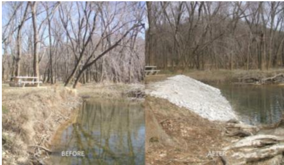
Figure 2.4: Pictures of streambank before and after completion of stabilization of project 42-54-00.
